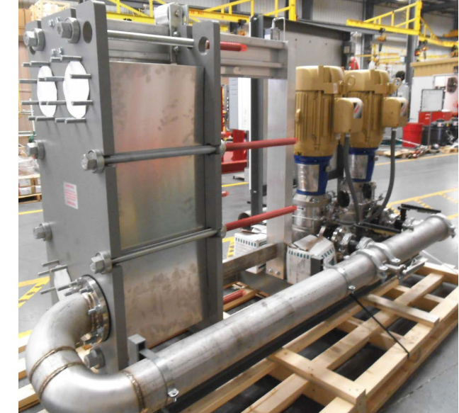
PROJECT: Pharmaceutical Plant
